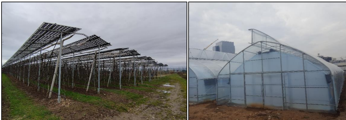
Figure 2. Left: Overhead agrivoltaic system with open sides, generating partial shade and solar electricity. Right: Greenhouse with semi-cylindrical roof and closed sides, with vents for climate control, adapted from (Akpenpuun et al., 2021).
