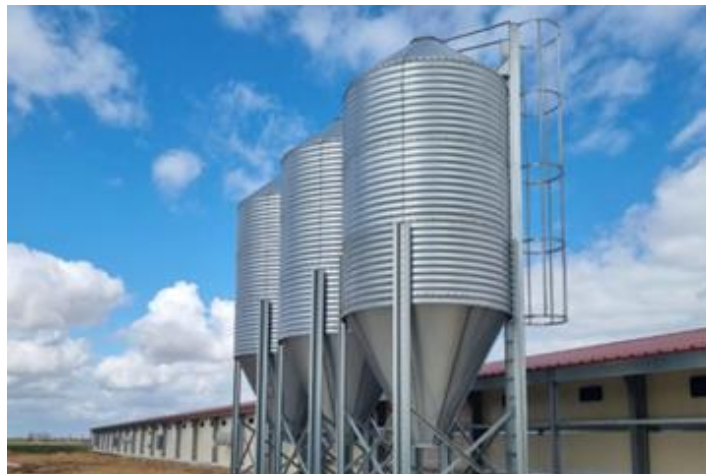
Figure 1. Corrugated silos in a livestock farm.
